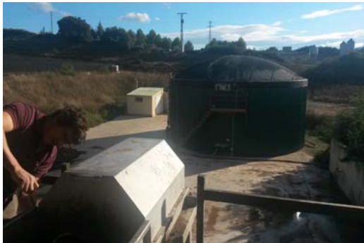
Courtesy: BIOVEC. Small-scale AD plant in Zaragoza (Spain)
